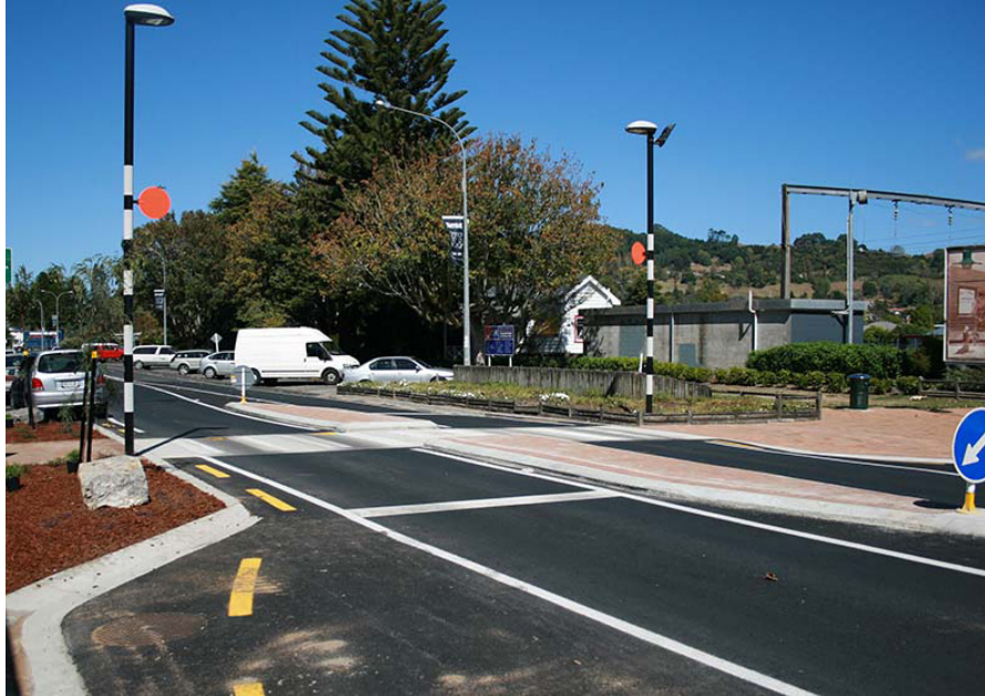
Rora Street roading renewal project.
