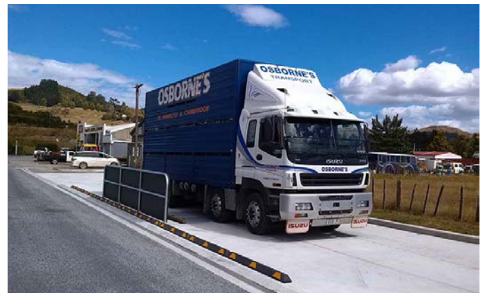
Stock truck effluent disposal facility - Te Kuiti.
