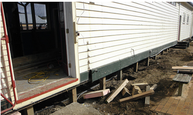
Replacement of the bearers - Railway Buildings.
