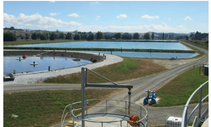
Te Kuiti Wastewater Treatment Plant.
